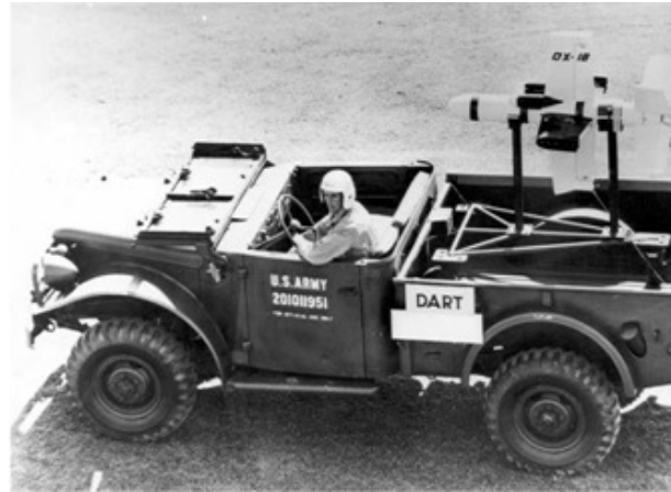
Figure 12. The Jeep mounted Dart prototype produced in 1958 (US Army photo).
