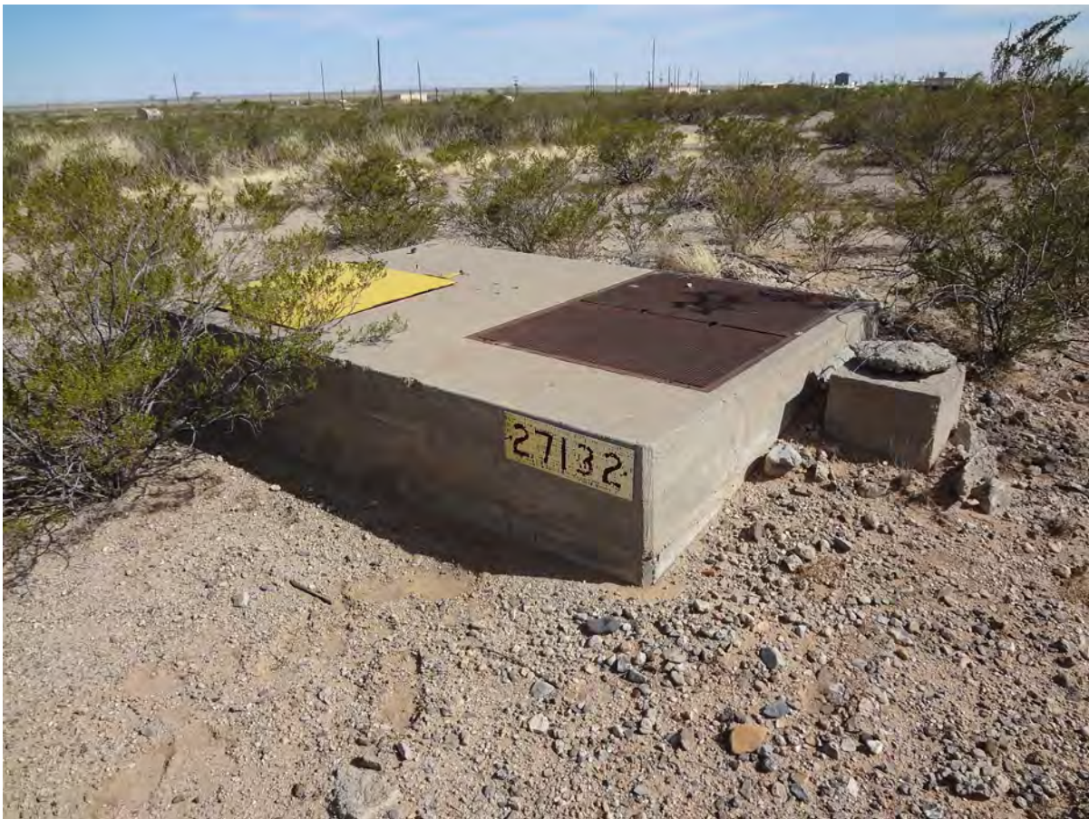
Figure 102. Property 27132, a good representative of the identical Fastax and Mitchell Camera Shelters installed at the SMR. View is to the southeast.
