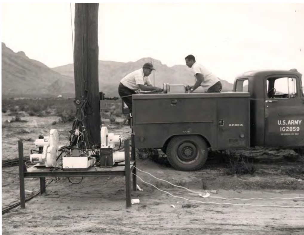
Figure 232. A camera is mounted on the "cart" that is winched to the boom at the top of the aerial camera suspension pole, circa 1950s ( undated photo on file at the WSMR Environmental Directorate ).
