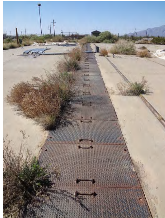
Figure 72. Property 27190, detail view of underground cable trench.
