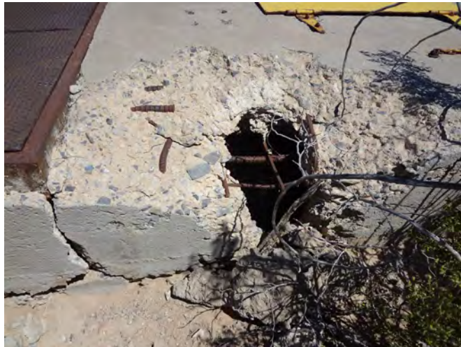
Figure 108. Property 27141, impact damage on south elevation.
