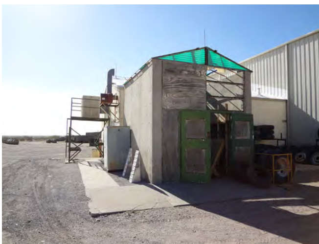
Figure 155. Modified concrete blast barricade, west elevation.
