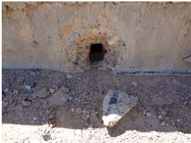
Figure 109. Property 27141, impact damage on north elevation.
