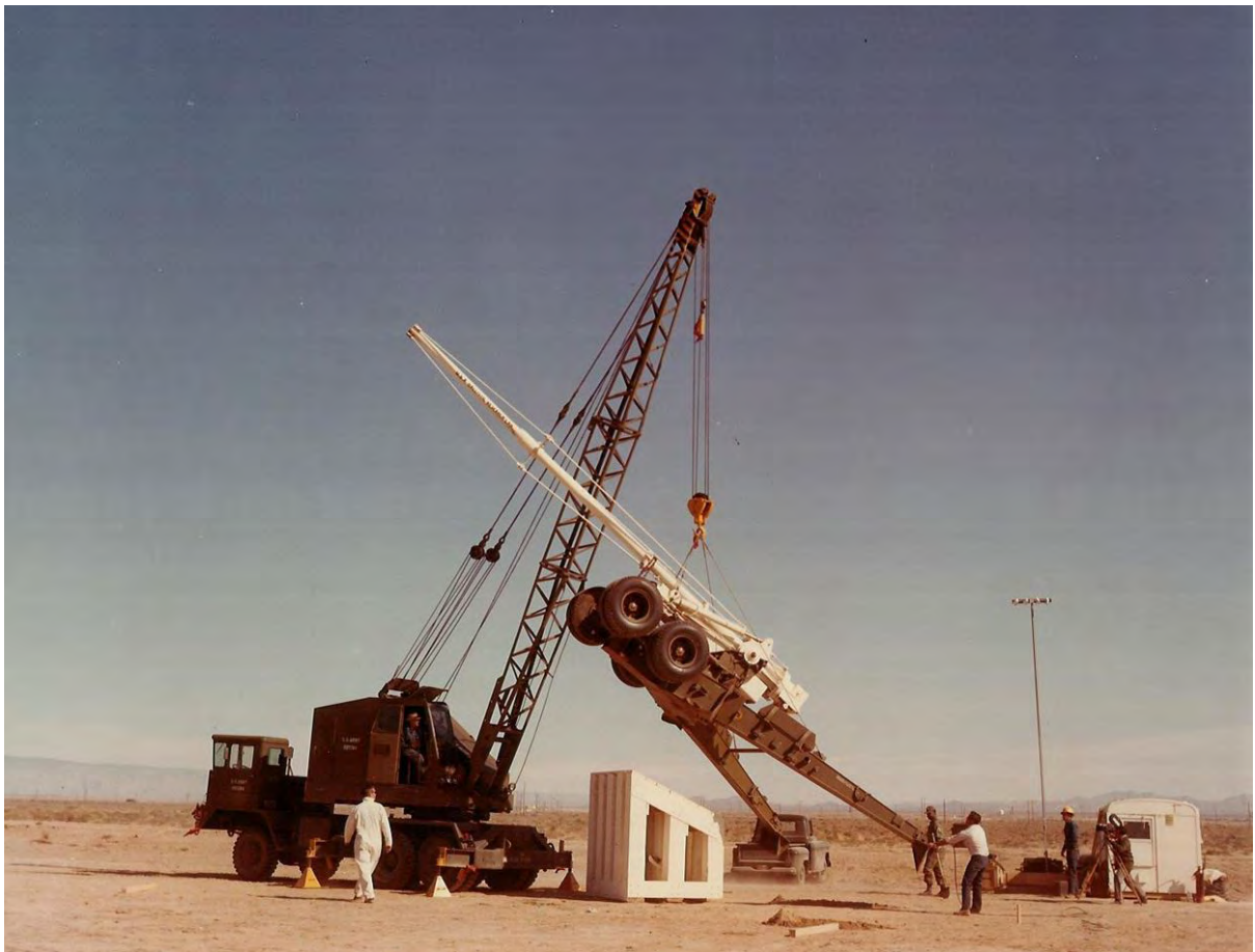
Figure 64. The 5-inch HARP gun being installed on the angled 45-degree platform at the SMR in 1965 (US Army photo).
