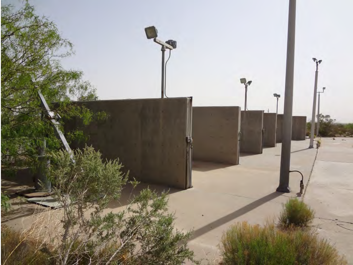
Figure 84. Concrete slab addition with concrete barricade walls on north side of original ASL launch pad, view to the northeast.
