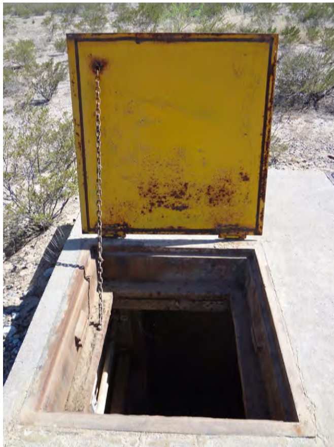
Figure 105. Typical Fastax/Mitchell Camera Shelter access hatch.
