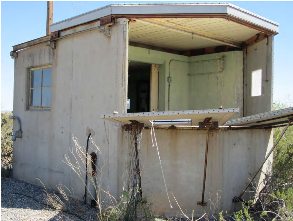
Figure 98. Property 27160, showing operation of folding panels on west elevation, view to the southwest.
