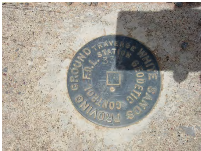
Figure 121. WSPG brass survey datum associated with Property 27175.
