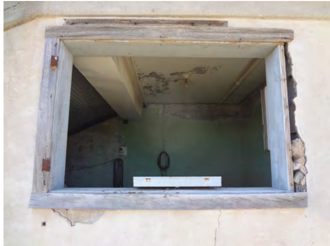
Figure 93. Modified window aperture of Property 27151.
