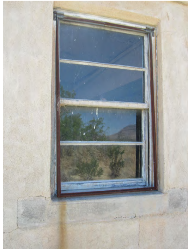
Figure 95. Detail of the double-hung steel window that is present in all the Bowen-Knapp Camera Shelters.
