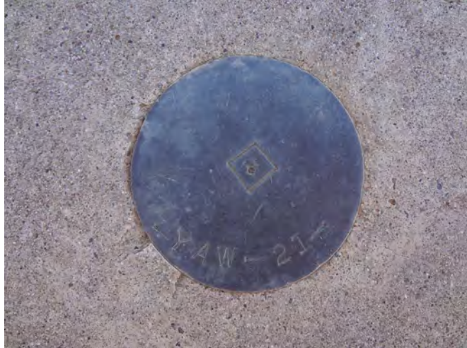
Figure 107. A typical “YAW” datum found at the southeast corner of each Fastax/Mitchell Shelter.
