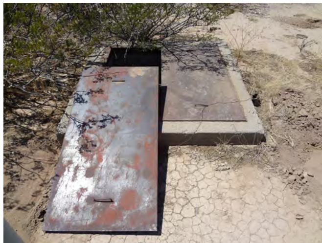
Figure 76. Property 27199, underground pull box.
