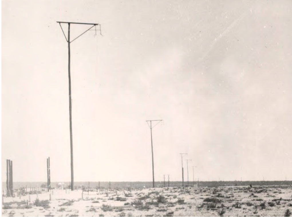
Figure 231. The series of aerial camera suspension poles along the SMR Yaw line, circa 1950s ( undated photo on file at WSMR Environmental Directorate ).
